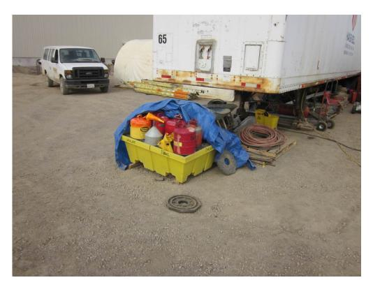
Photo 5: Secondary containment provided for fuel tanks at the Compressor Station site.
