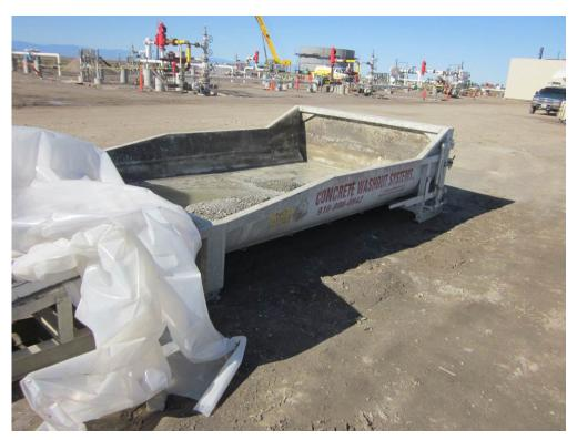
**Photo 3:** Concrete washout provided at the Compressor Station site for containment of excess concrete.
