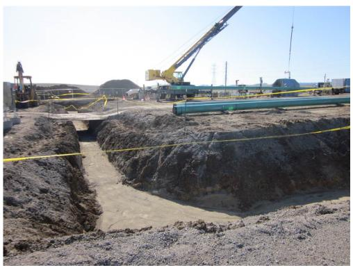
**Photo 6:** Trenching is underway at the Metering Station site for natural gas pipeline connection.
