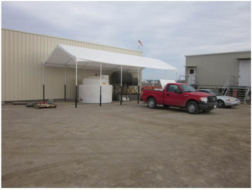
**Photo 4:** Liquid hazardous materials storage at the Compressor Station site observed to have adequate secondary containment and a cover to prevent rainfall collection in the secondary containment tank.
